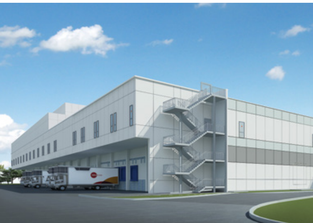
SATS Inflight Catering Centre 2 is undergoing an $18 million expansion to increase our total aviation production capacity in Singapore to 115,000 meals a day.
